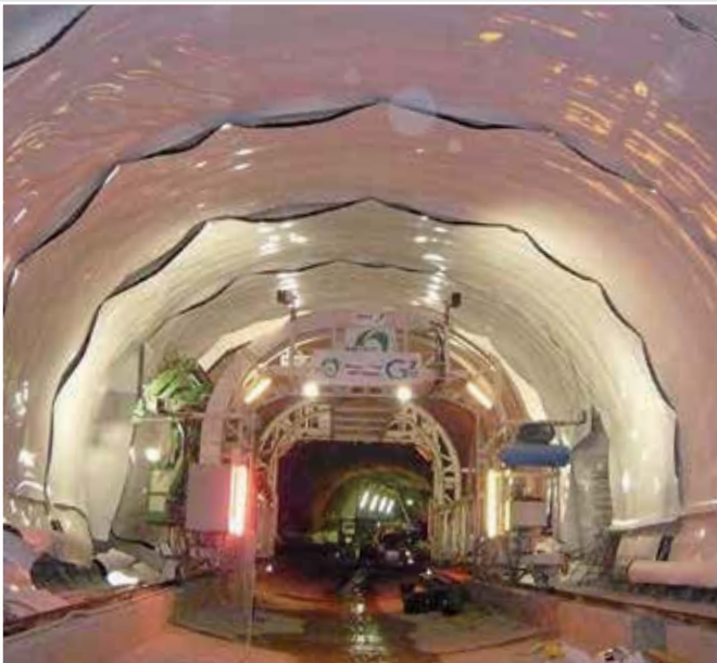
Tunnel PVC 2.5 mm
