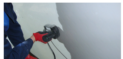
Induktofix welding disc for AGRU liner
